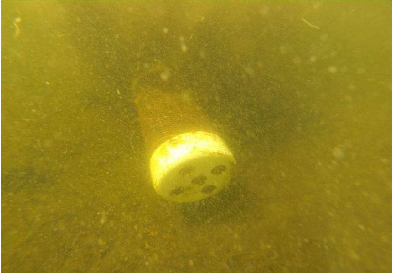
Screen on Inlet Pipe
