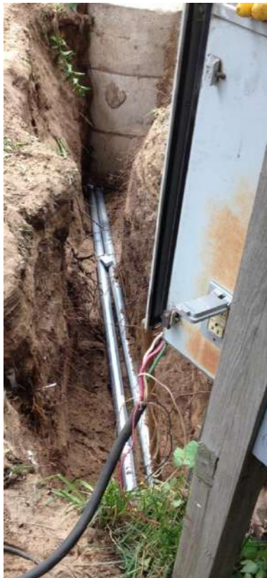
New conduit to control panel.
