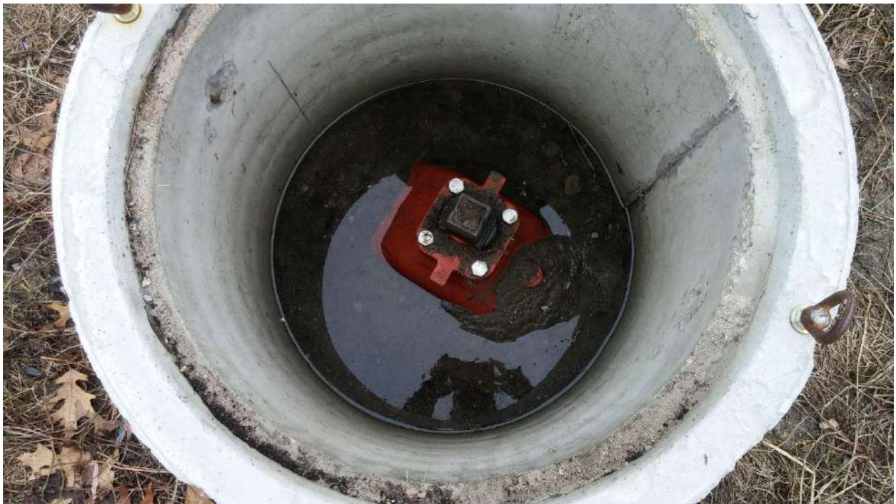
Inlet Pipe Valve Chamber Interior
