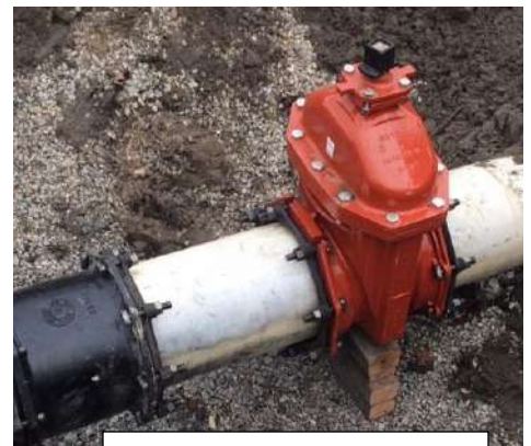
New valve on intake pipe
