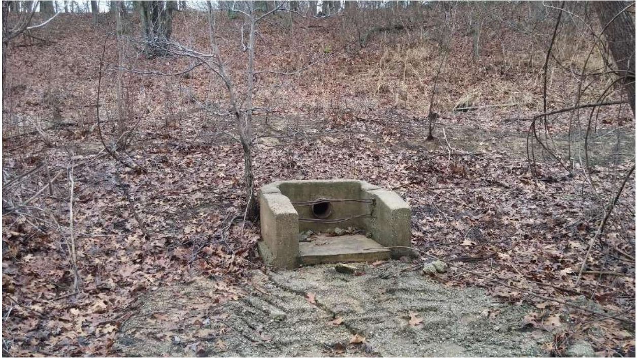
Outfall at Infiltration Basin
