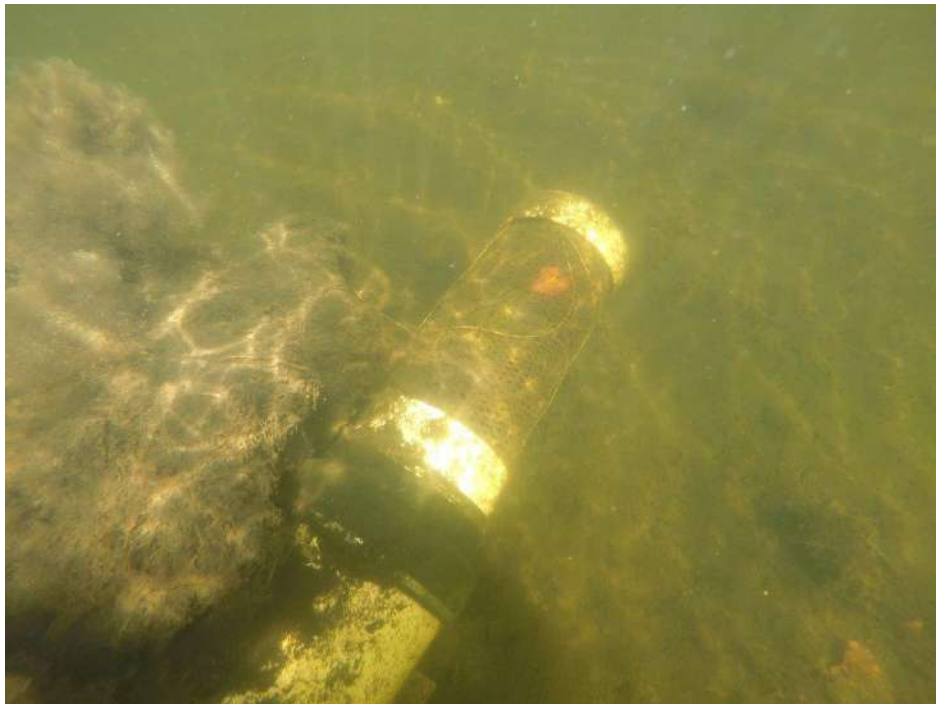
Screen on Inlet Pipe
