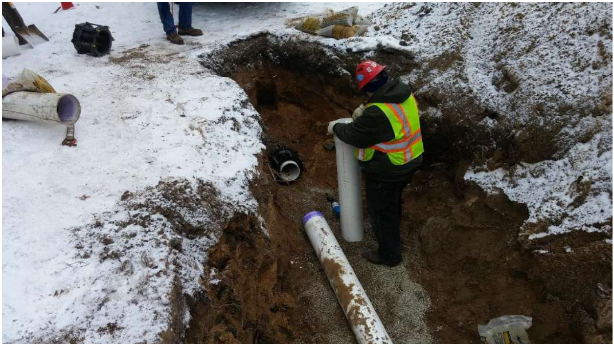
Force Main Pipe Repair – February 4, 2016
