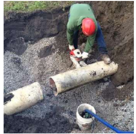
Fixing broken intake
