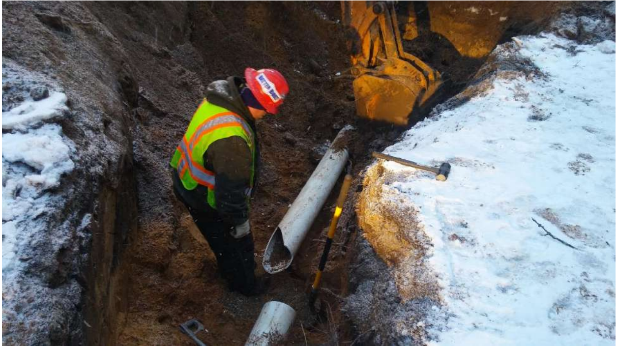
Force Main Pipe Repair – February 4, 2016
